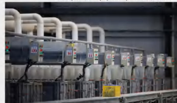
Charging process 充电工序
